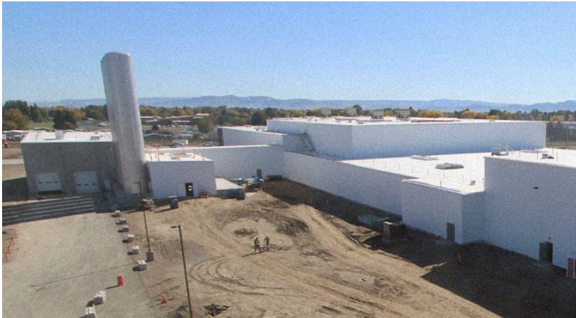
The Suntado, LLC facility under construction in Burley, Idaho.
